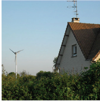
Generating power for property in France (3)
